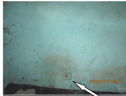
FIG 7: East side wall showing pock mark of bullet shrapnel and blood smudge on wall from which scrapings were taken
