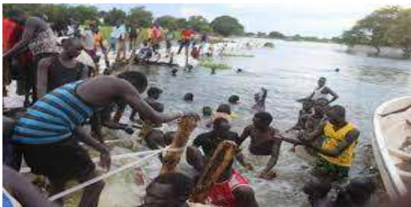
Youth Repairing broken parts of dykes between kolmarek and jalle
