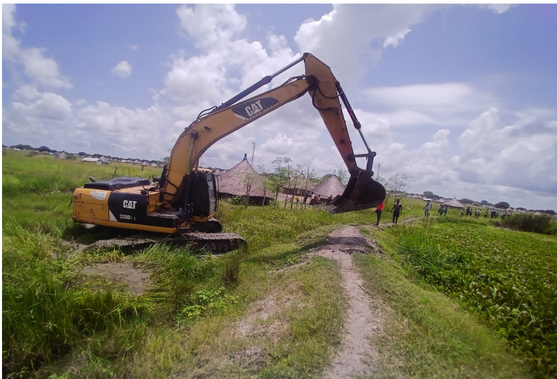
Actual work begins on the 12.7 Kilometers Secondary dyke
