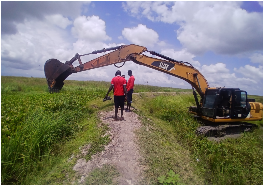
Youth members standing on the renovated part in Panyagoor
